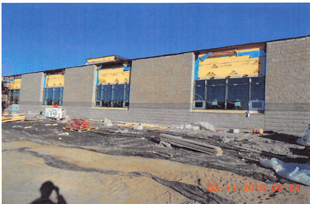
Exterior Veneer completed / glazing installed
