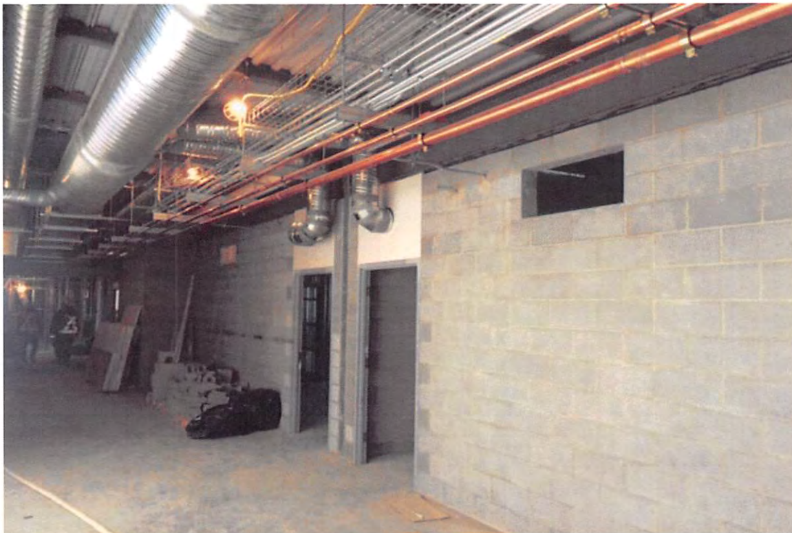
South Wing Mechanical Rough-ins
