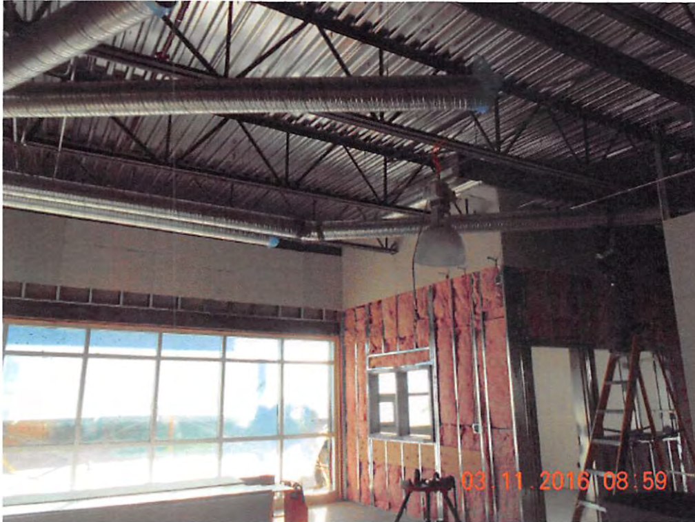
Interior dry walling / Duct work installation
