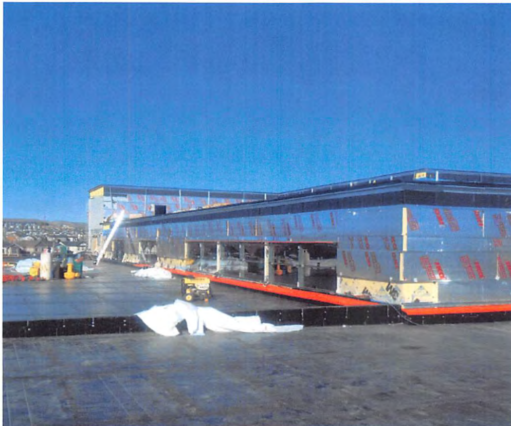
Roofing ongoing / Insulation being installed
