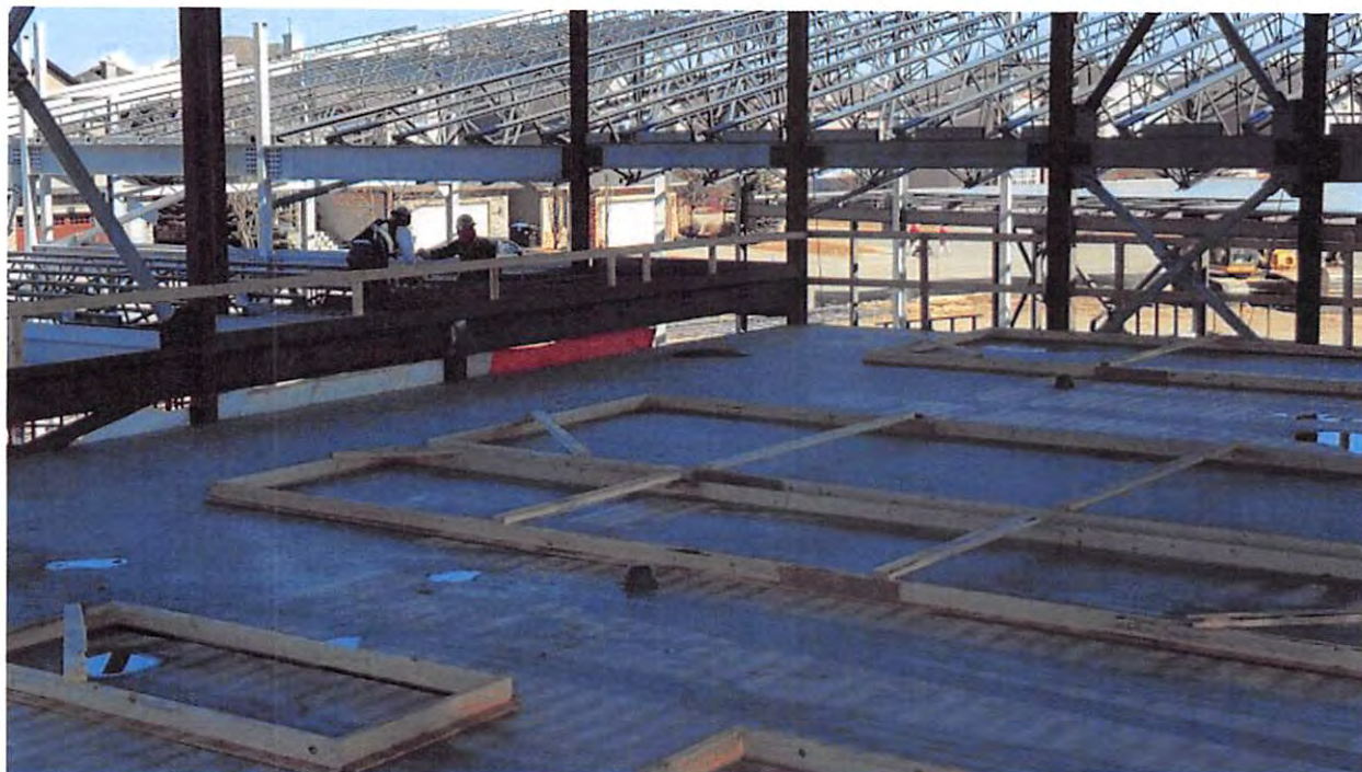
Steel bridging Northwing
