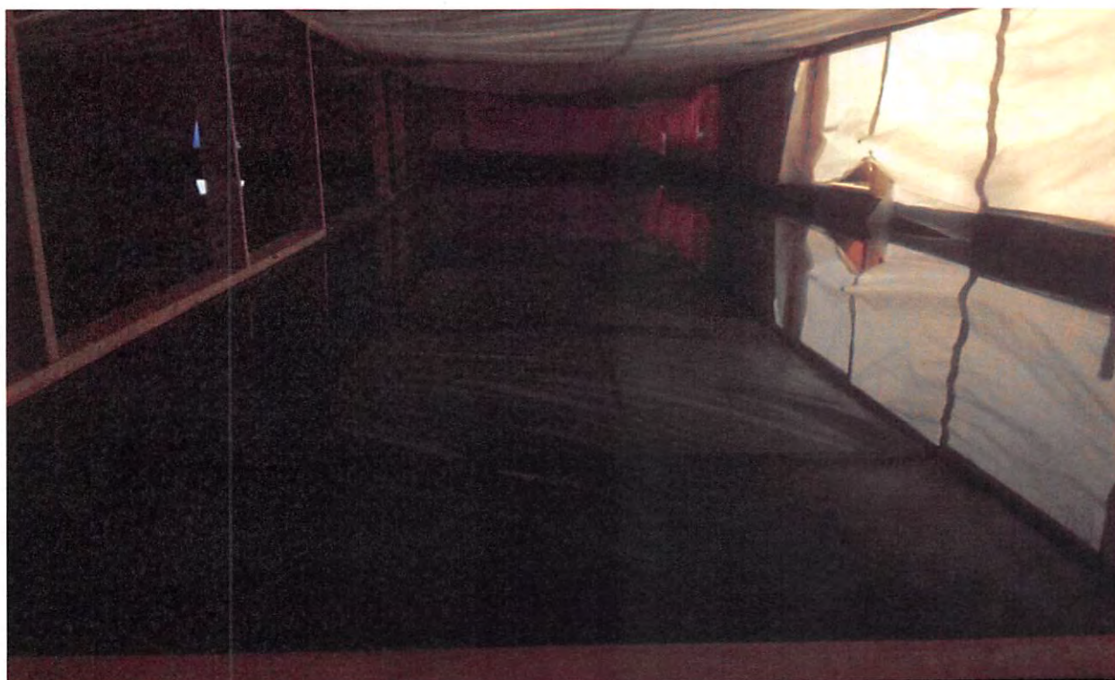
Pool: filled for Testing
