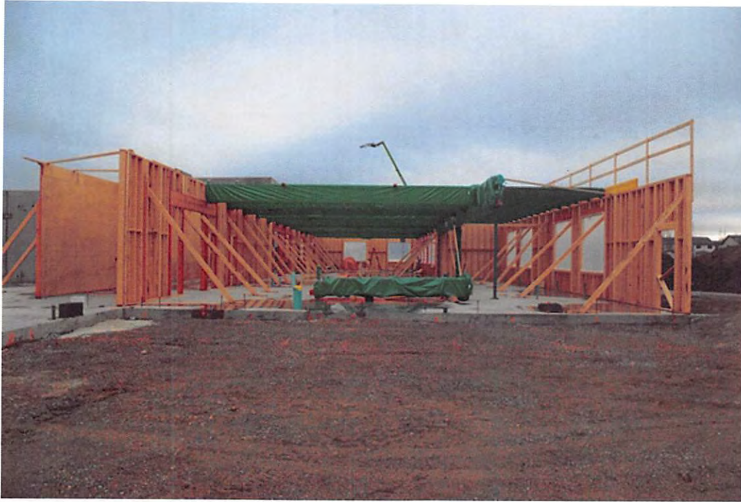
Bldg 2 Classroom Glulam
