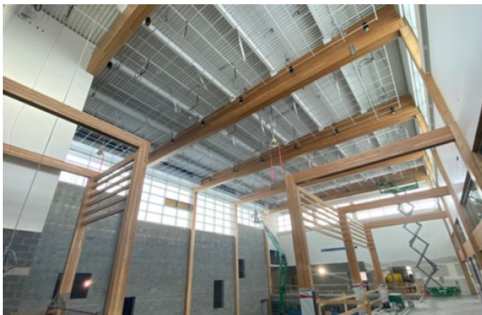
Gathering Space – 2 nd floor balcony
