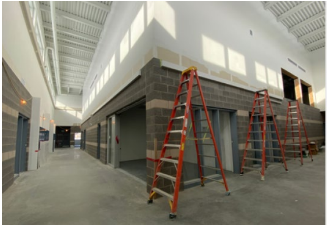
2nd Floor hallway – classroom wing
