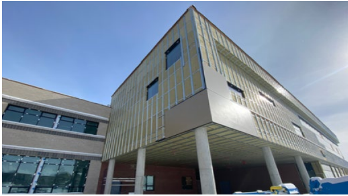
West Elevation – Library & entrance
